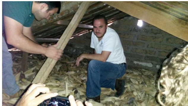
Attic on top of kitchen or room
