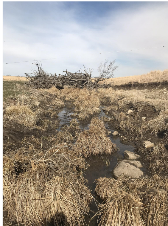
Figure 9: The dam at site 3
