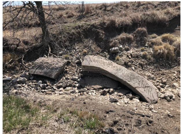
Image 8 & 9: Slump and undercut erosion with two concrete slabs placed by landowner to slow flow at site A-3. Left slab is 1.2 m and right slab is 2.85 m.
