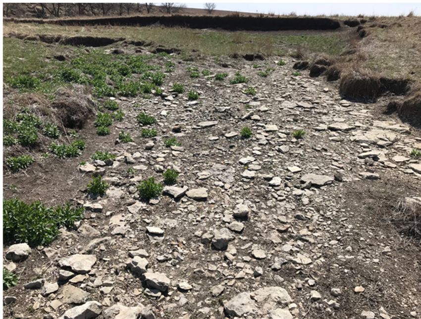
Image 6: Site A-1. Downstream look at steep cut bank exposed at the horizon of the picture. Tabular blocks at stream bottom.
