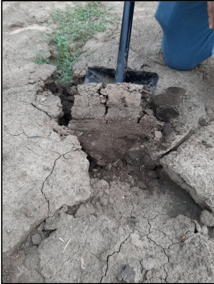
(Figure 5.1.1): Eroded Soil Profile
