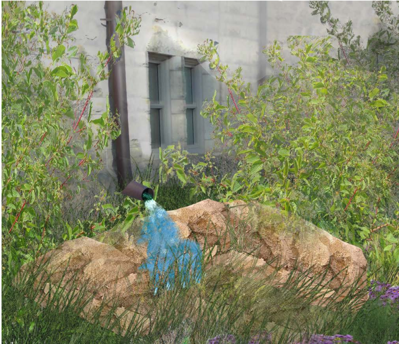
DISCONNECTED DOWNSPOUT WITH LIMESTONE LEVEL SPREADER
