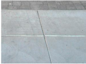
V-Cut Saw Joints
