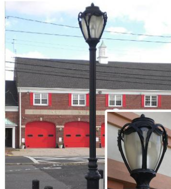
Sentry Central Park Light Fixture - 17th St. Claflin
