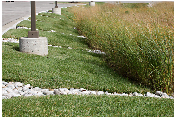
STORMWATER BMP AT PARKING LOT EDGE; LENEXA, KANSAS
