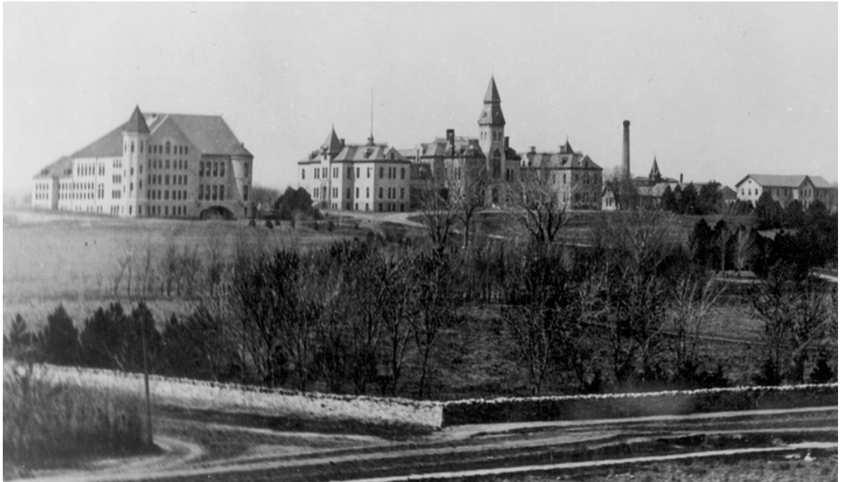
THE CORNER OF ANDERSON AVENUE AND NORTH MANHATTAN AVENUE, POST 1885
