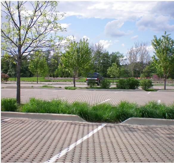
PERVIOUS PAVEMENT PARKING; CHICAGO, ILLINOIS
