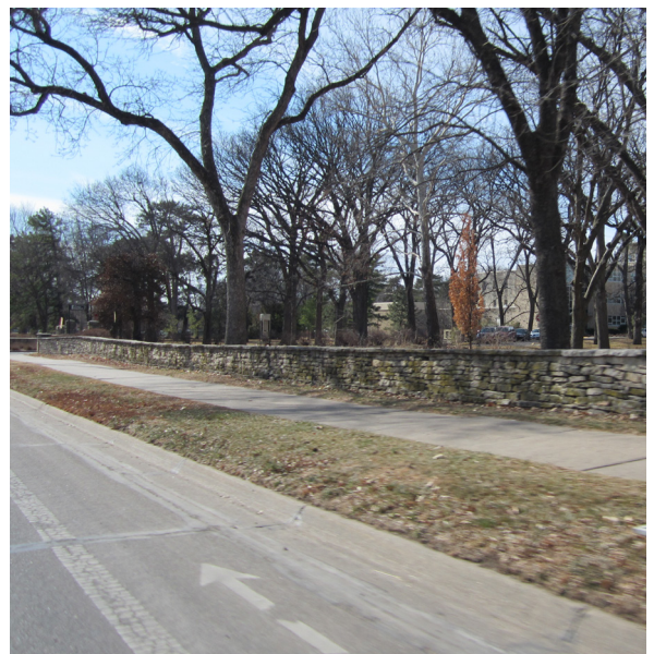
HISTORIC BOUNDARY WALL ON N. MANHATTAN AVENUE
