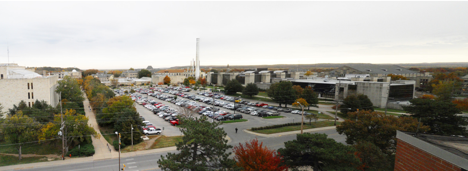
EXISTING VIEW OF CAMPUS LOOKING SOUTHEAST FROM DENISON AVENUE.
