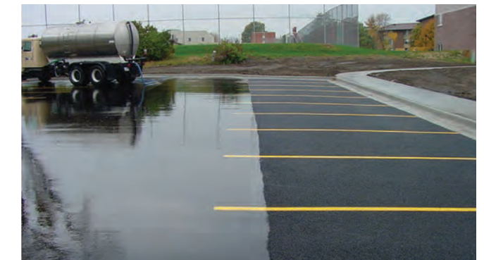
Example Permeable Pavement
